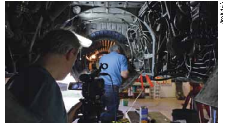
▲ Filming Dave Yates, one of the propulsion team, fitting a fire extinguisher in the lower engine bay in November 2011 with the Canon 105
